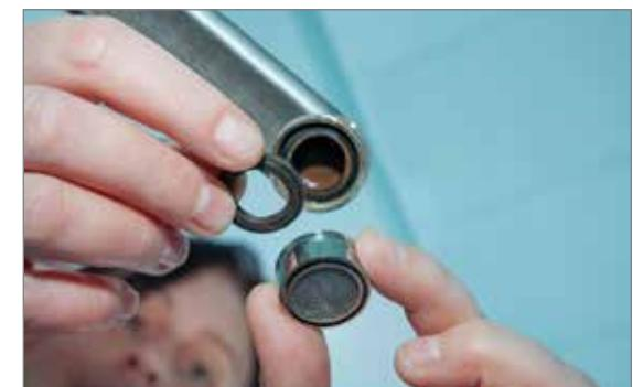
■ Clean Aerators—Aerators are small attachments at the tips of faucets which regulate the flow of water. They can accumulate small particles of lead in their screens. It's a good idea to remove your aerators at least monthly and clean them out.
